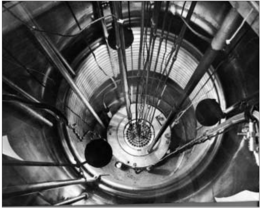
Fig. 7. Looking down into the pool of the original 10-kW TRIGA Mark I reactor at San Diego, Calif.
