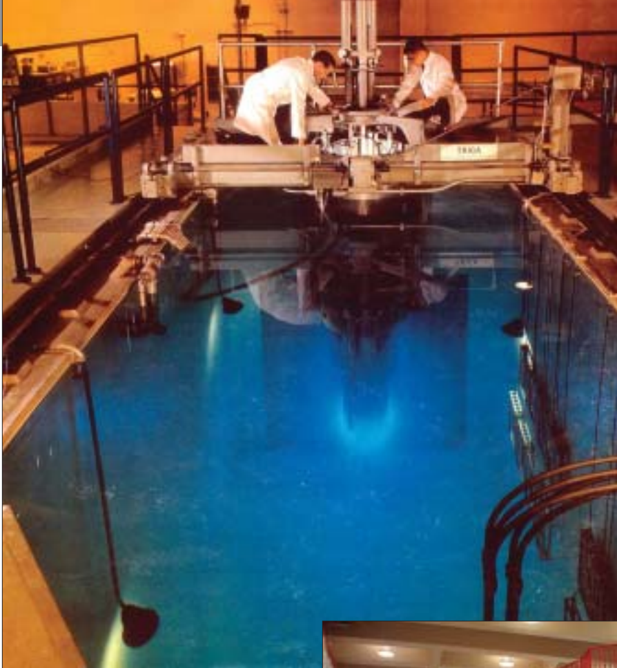
Fig. 14. TRIGA movable core reactor at Northrop Corp., in California
